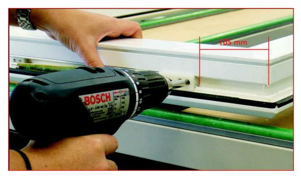
2. Position the striker plate behind the bead groove on the outer frame 45mm from the corner and screw into position.
