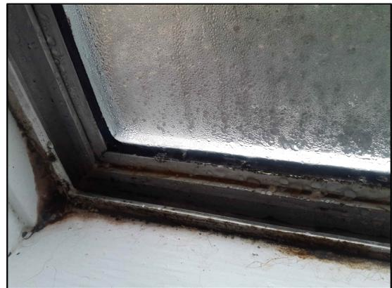
*Condensation will regularly form on cold internal surfaces, causing mould, risking health and damaging the building fabric.*
